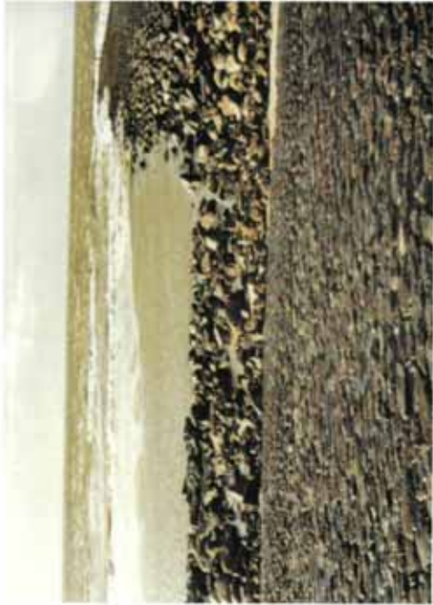
Fig. 4.30 Bestorting
